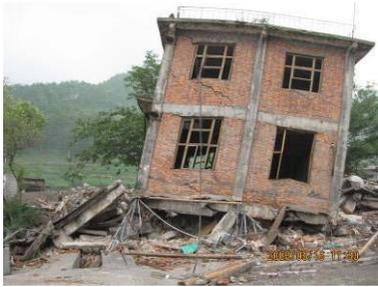
A gas station using masonry structure with bottom RC frame, Hongbai
