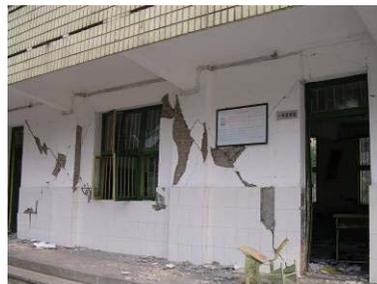
Severe damage in the load-bearing walls and columns of the teaching building of Huayuan St. Middle School, Jiangyou
