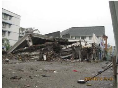
Collapse of a RC frame with a heavy roof, Dujiangyan
