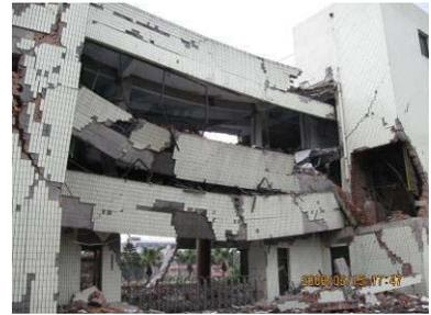
Fig.3 Seismic damage of RC frame-masonry hybrid structures
