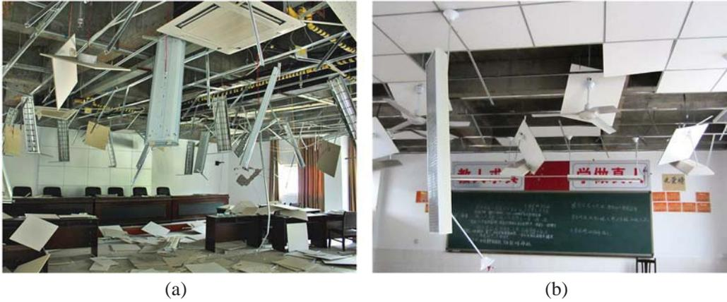
Fig. 4 Collapse ceilings in (a) the main meeting room of Lushan Radio and TV Center and (b) a classroom in Gaohe Middle School, Qionglai.
