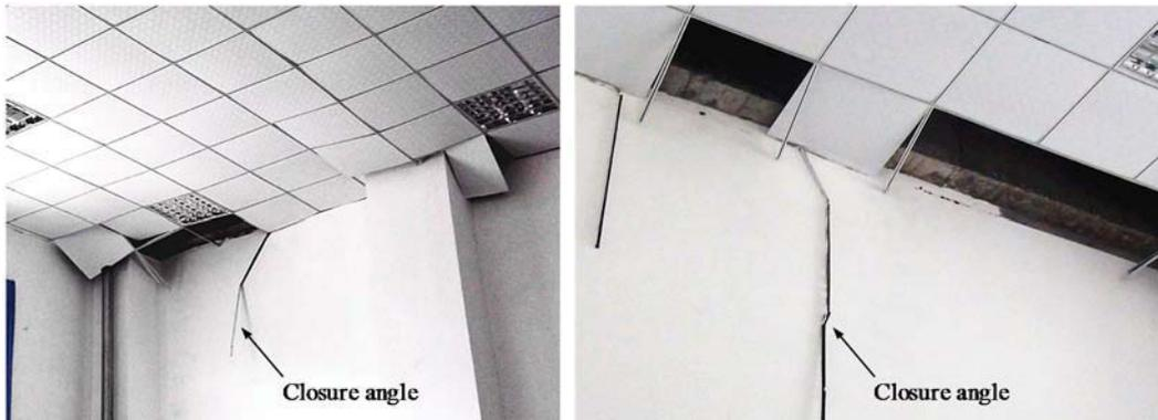
Fig. 5 Dislocated closure angles in Daxing Middle School, Ya'an.
